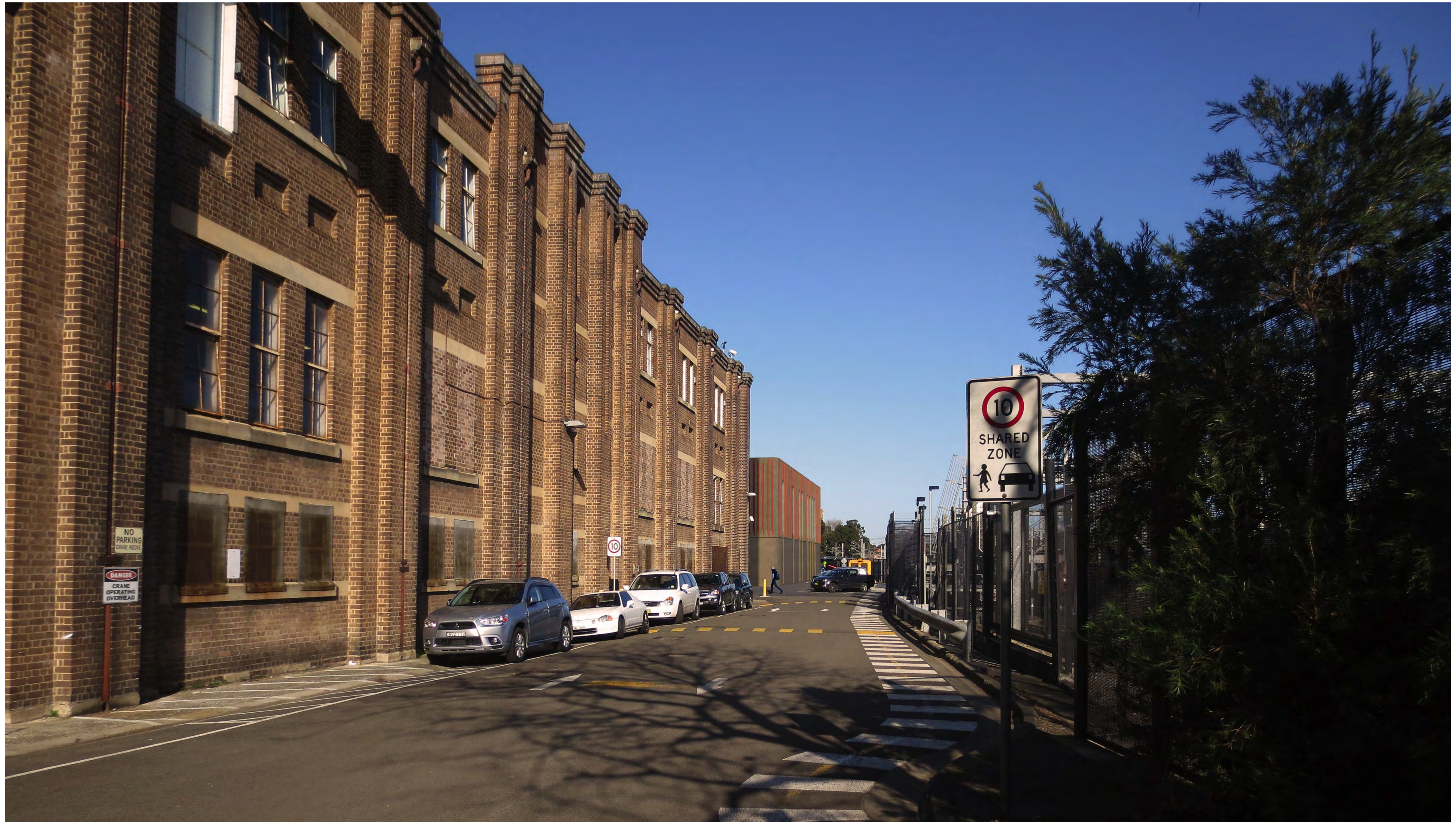
1 VIEW FROM NORTH
