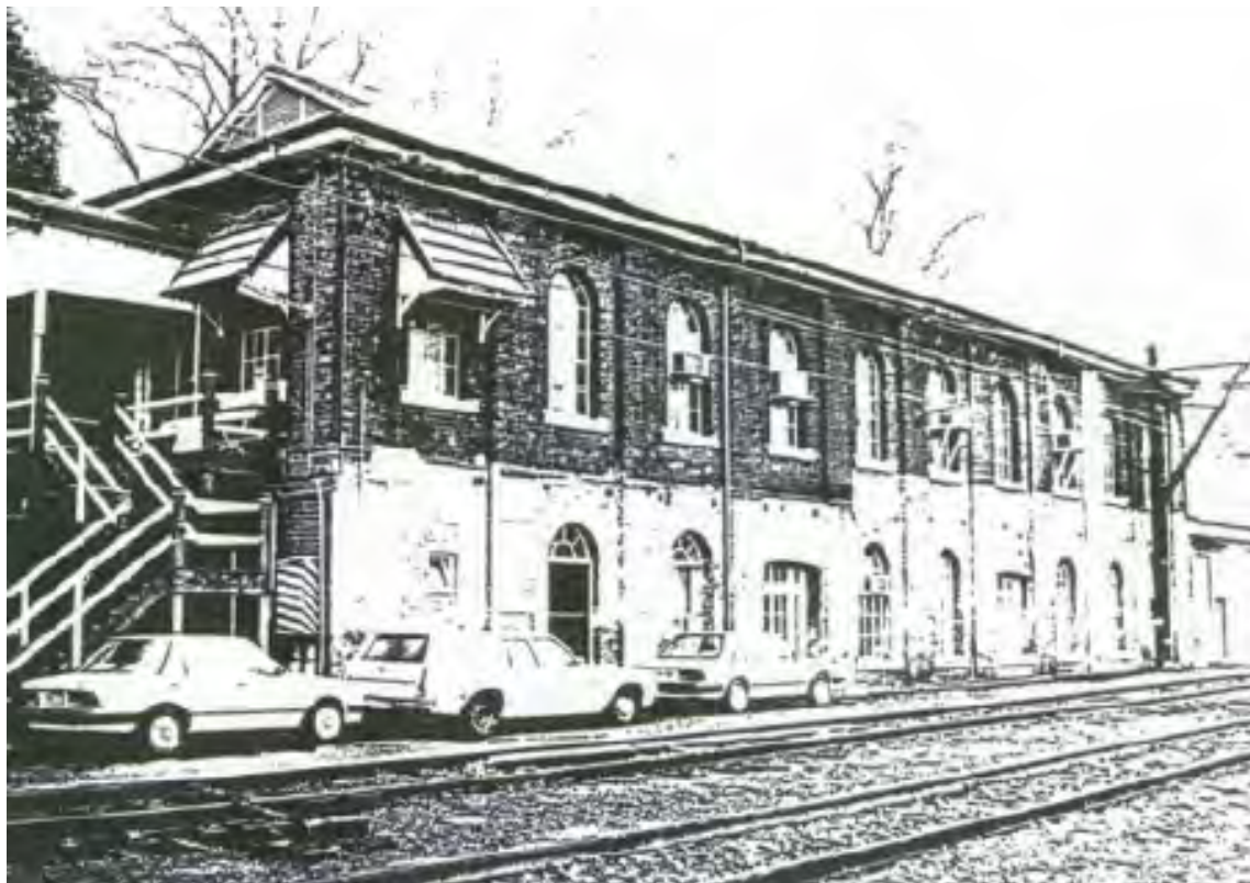
Figure 19: Carpenters Workshop (now demolished) circa late 20 th century. Source: Sheedy, Sydney Yard Conservation Plan , 1988.
