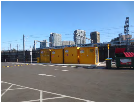
Figure 52: Hazard materials storage in containers located on northern boundary.
