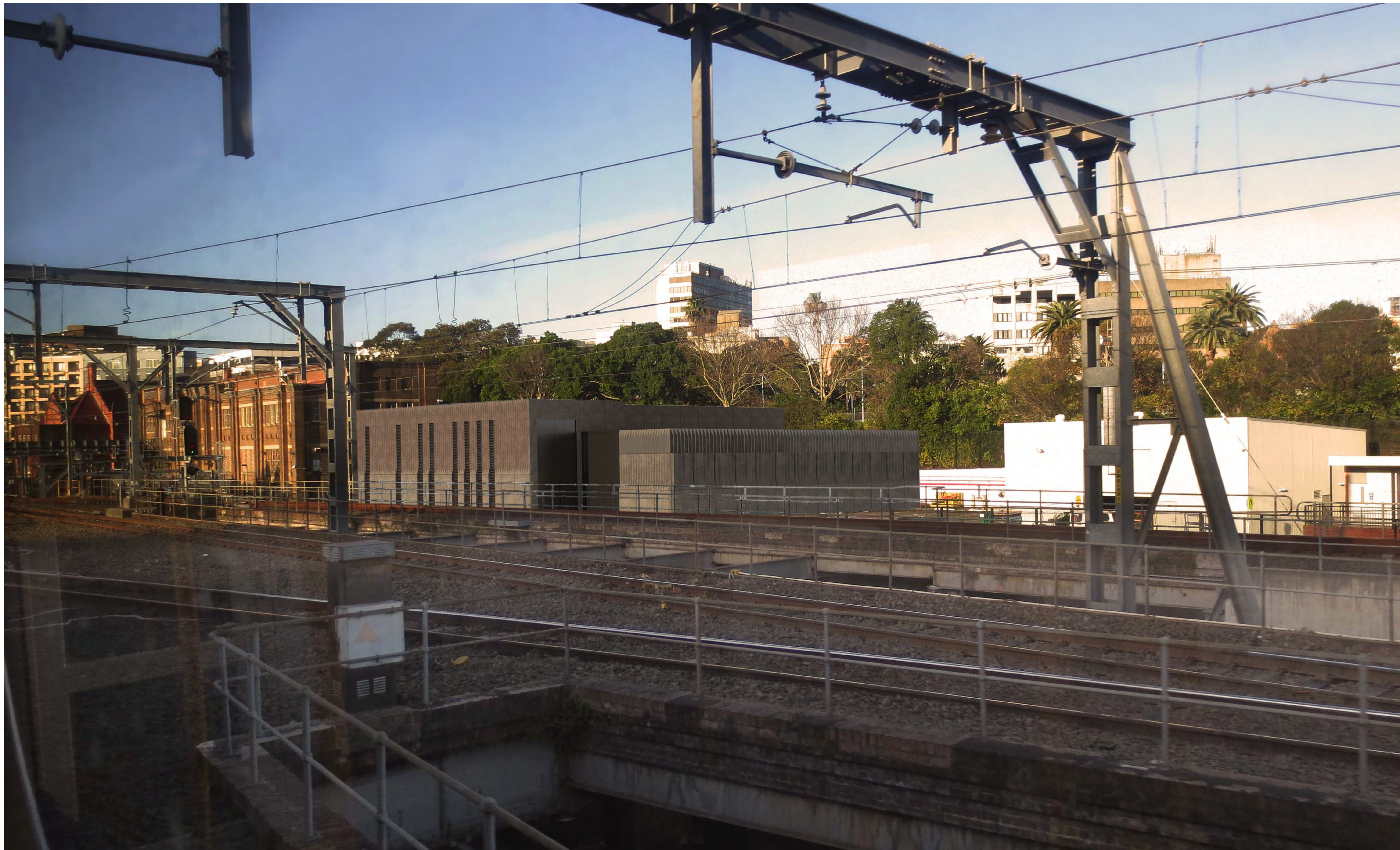
1 VIEW FROM RAIL CORRIDOR
