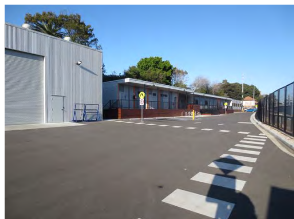
Figure 49: View southeast towards maintenance facility and office demountable buildings.
