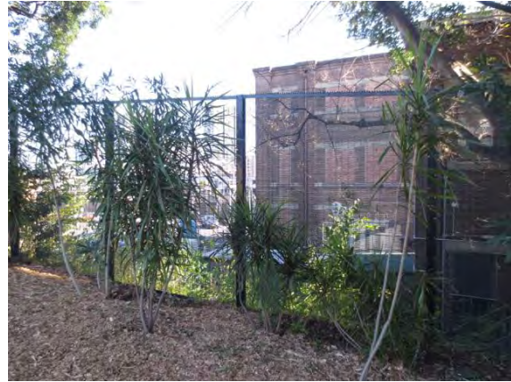
Figure 33: Looking west into site from Prince Alfred Park. Prince Alfred Substation is in view.
