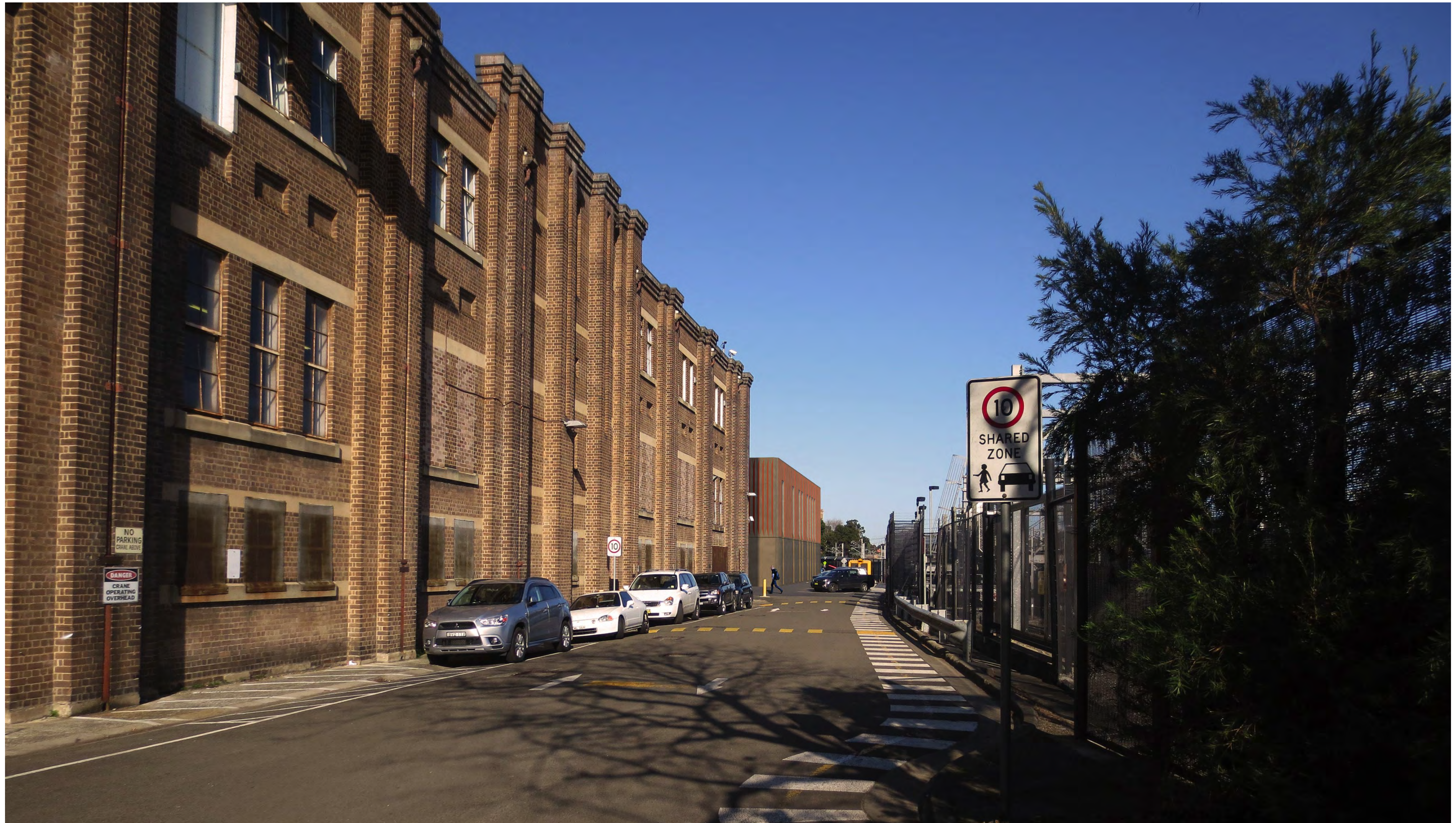
1 VIEW FROM NORTH
