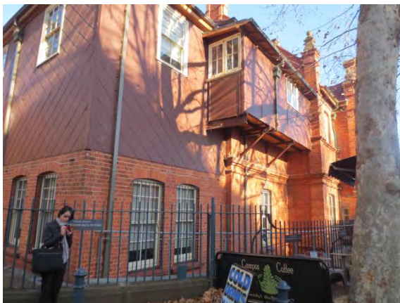
Figure 24: Southeast corner elevation of former Railway Institute Building taken from Chalmers Street.
