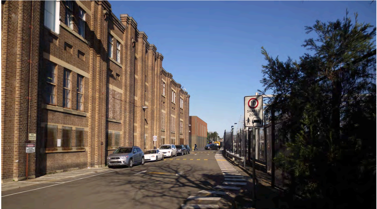
Figure 60: View from access road looking south past Prince Alfred Substation. TZG, 2015
