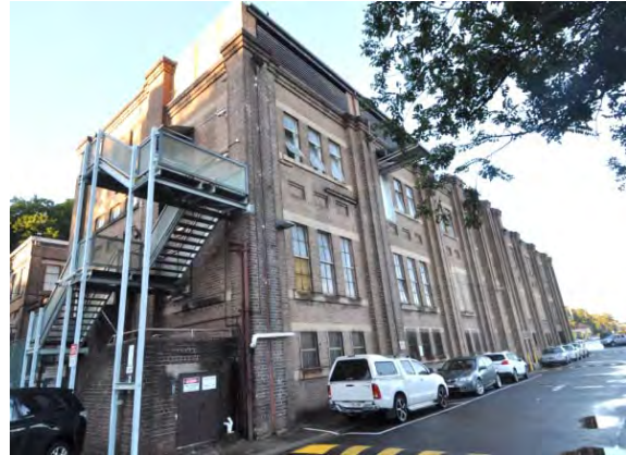
Figure 45: North west elevation. Pump well doors under stairs on left side.
