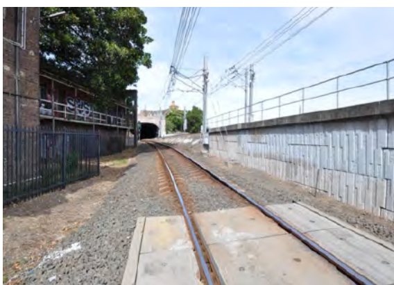
Figure 54: View of Airport Line and tunnel showing its close proximity to the Draughtsman's Office to left.
