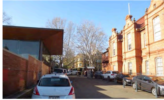
Figure 27: View east from site access road. Former Railway Institute Building is on right.
