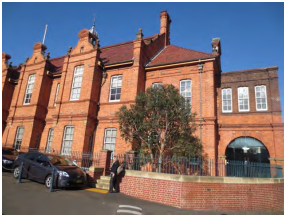
Figure 34: South elevation of former Railway Institute Building.
