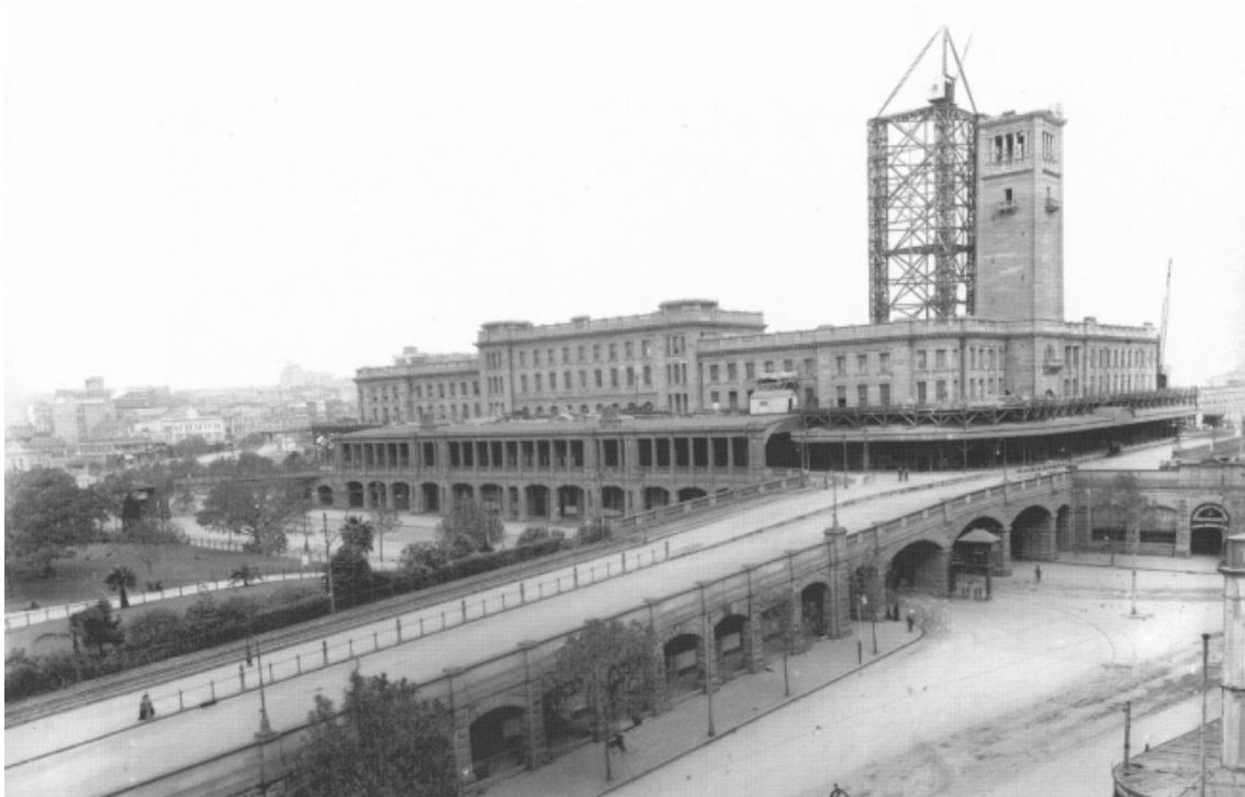
Figure 13: The clock tower under construction. Source: Oakes, Central , p31.
