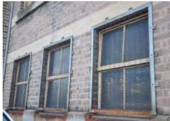
Figure 47: Ground floor windows with security mesh over.
