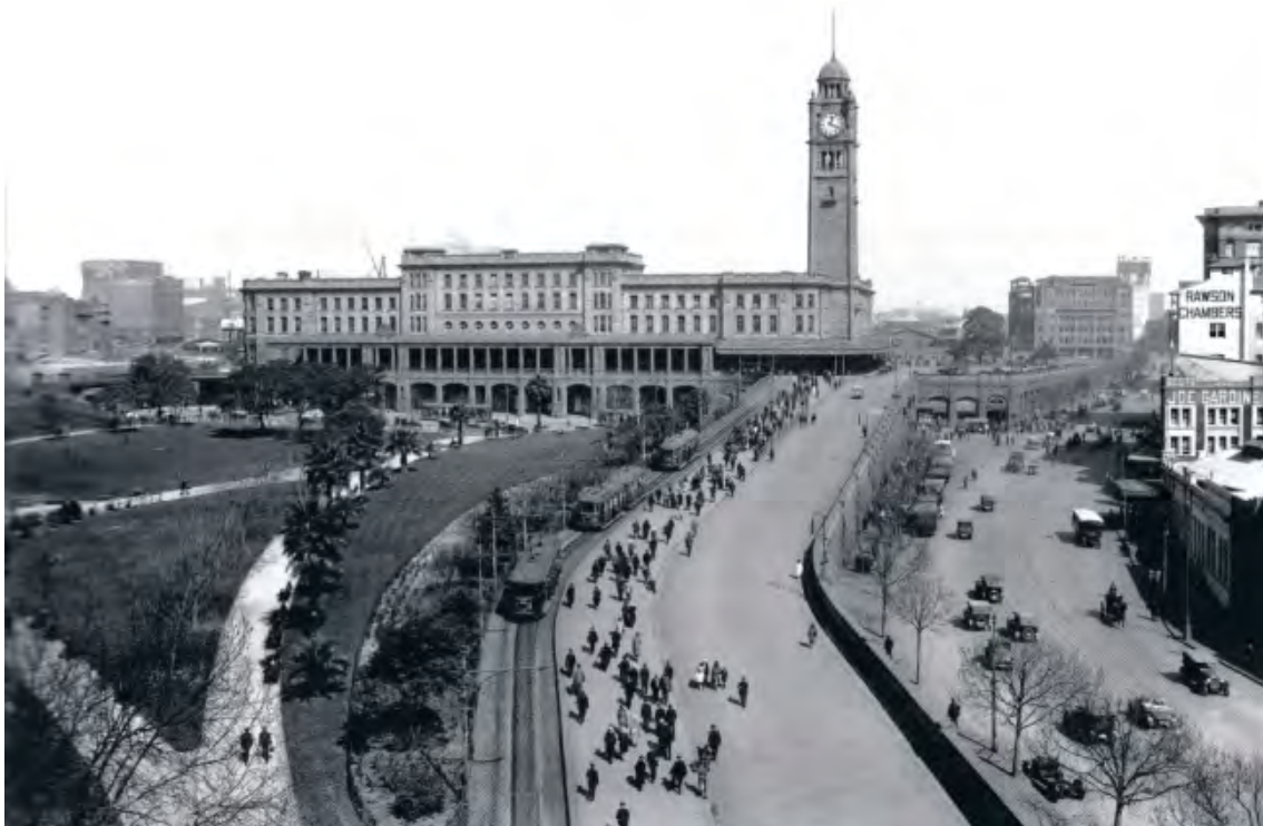
Figure 14: The completed Station, with the west tram ramp in the foreground, 1924. Souce: McKillop, Century of Central , p45.
