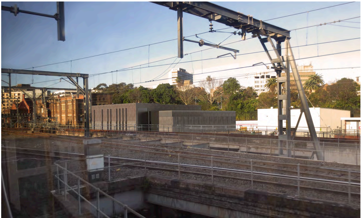
Figure 61: View from the rail corridor looking north east. TZG, 2015
