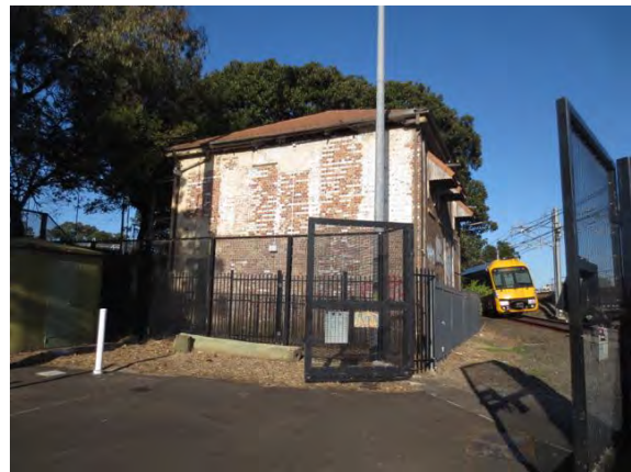
Figure 53: Former Engineer's Office and Draughtsman Office located beyond fence at southern end of the Prince Alfred Sidings.
