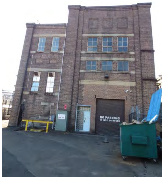
Figure 42: South elevation of Prince Alfred Substation.
