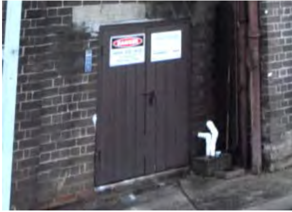
Figure 44: Detail of Pump Well doors.
