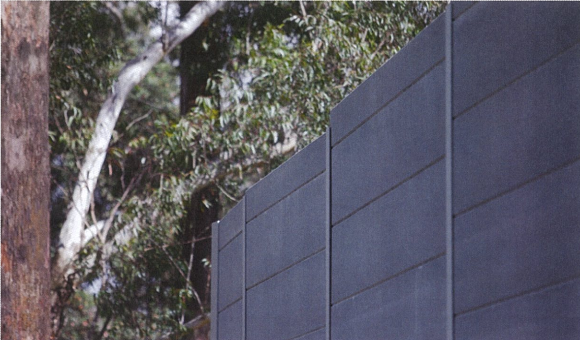
Figure 6 - Hebel Wall Noise Barrier at the Cheltenham Services Facility Site
