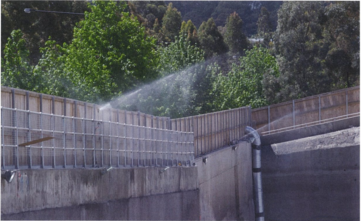
Figure 11 - Dust Mitigation at Norwest Station Site
