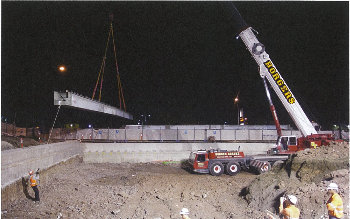
Figure 9 - Sydney Monorail Beams being re-used at the Norwest Station Site
